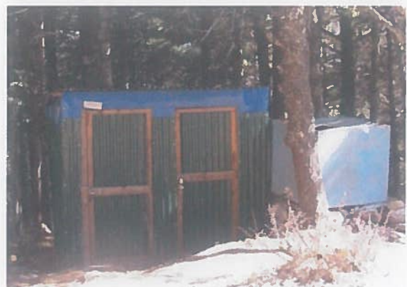
Figure 8: Drinking water and toilets built in Safe Evacuation center, Phungithanka
