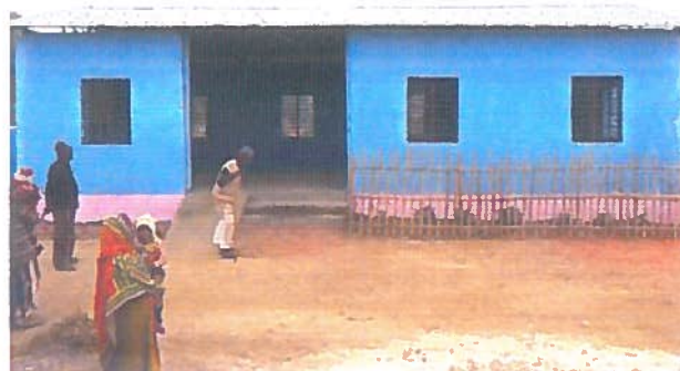
Figure 11: Evacuation center built in Nainhi, Mahottari
