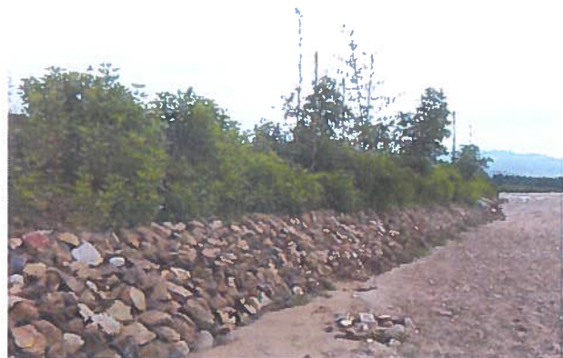
Figure 5: A stretch of embankment after the bioengineering works in Hadiya, Udayapur
