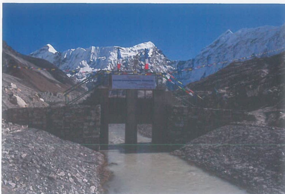
Figure 1 Imja Lake lowering structures -open channel with regulatory gate, constructed to drain water from the Lake
