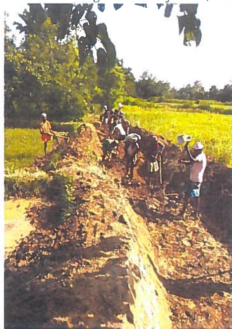
Figure 9: Community engaged in construction of FPDS, Nainhi, Mahottari
